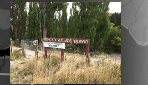
Wetland signage is out of date and in need of revitalising. Corten steel signage will replace this whilst maintaining a rustic aesthetic seamless to the surrounding landscape.
