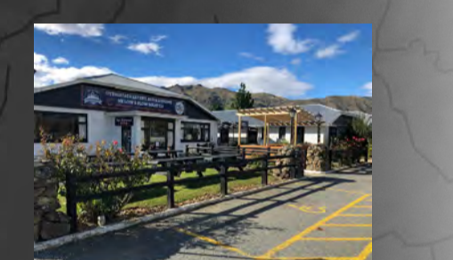
Otematata bar and hotel using a combination of hardwood and greywacke rocks.
