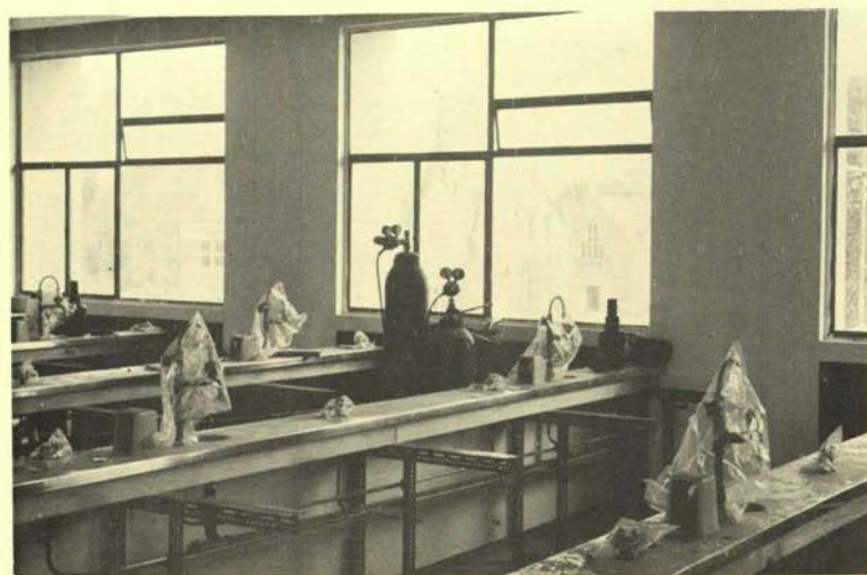
INSTALLING LABORATORY EQUIPMENT IN THE HILGENDORF WING
